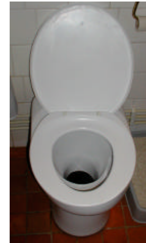
Figure 8. Example of a urine-diverting toilet with dry handling of faeces.
